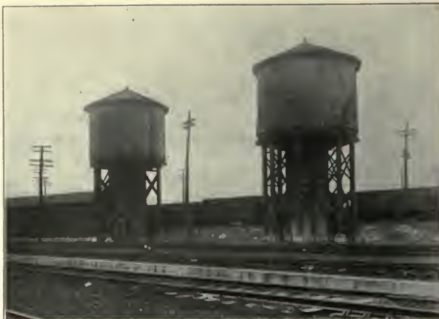
FIG. 657. FACILITIES TO BE ABANDONED. Water tanks of the Lake Shore & Michigan Southern Railway at 63d Street and Michigan Avenue. These tanks are of wooden construction throughout. In the event of electrification, they will be rendered worthless to the railroad in their present location. Owing to the necessities of operation during construction it will not be possible to transfer them to a new location until the need for similar facilities elsewhere has been met. They are, therefore, regarded as property to be abandoned.
